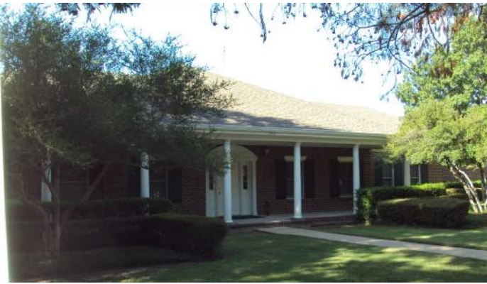
Celestial Road Pump Station
